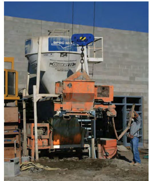
— Grout Hog crane bale system in use.
