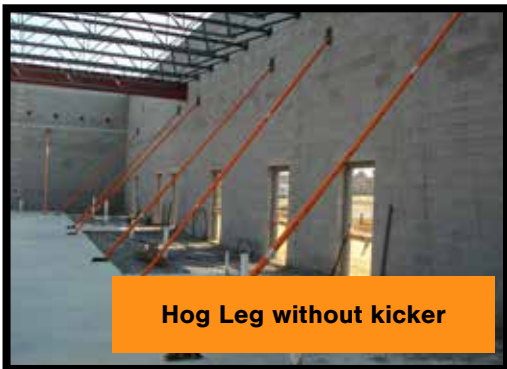
Same brackets attach at anchor location
