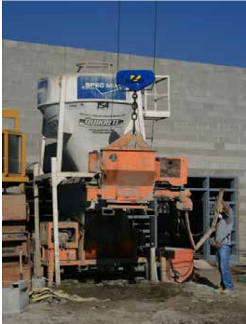
Grout Hog crane bale system in use.
