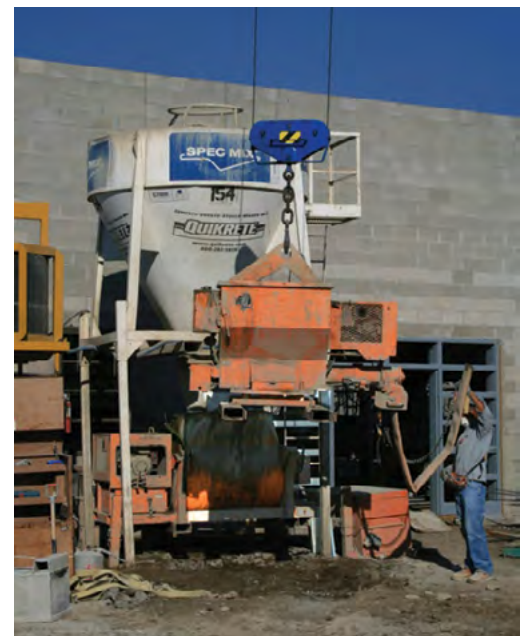
— Grout Hog crane bale system in use.
